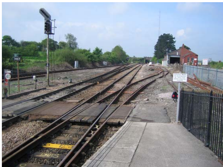
Disabled access to & from platforms 2 & 3
